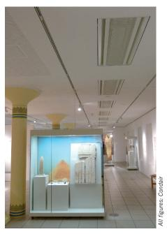
Figure 7 The outside air previously pre-tempered and humidified in the HVAC units is mixed with room air in the ceiling induction units, cooled in a water heat exchanger and then enters the exhibition rooms as supply air
