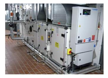
Figure 5 Two central air conditioning units with air outputs of 7,500 m<sup>3</sup>/h each were installed on the roof of the museum. On the top left is one of the two gaspowered Condair steam humidifiers
